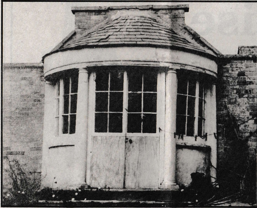
■ At the centre of a planning row... the 19th century gazebo, before to its demolition.
