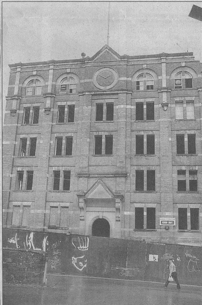
■ IN PROGRESS: The work is in hand to convert the old Hill Paul clothing factory to flats.
