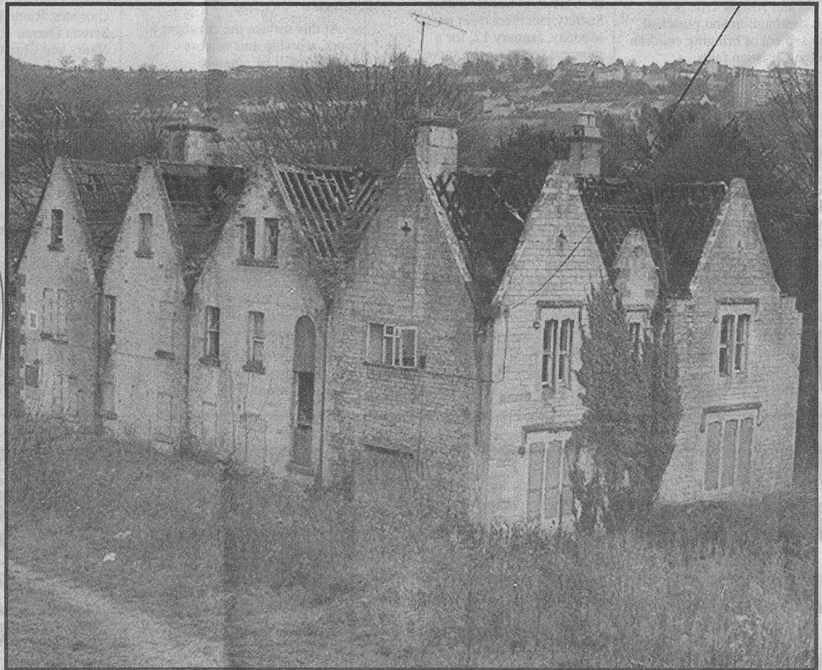
■ Derelict Uplands House will no longer be turned into a home for 75 old people after vandalism left the building in a poor state.
