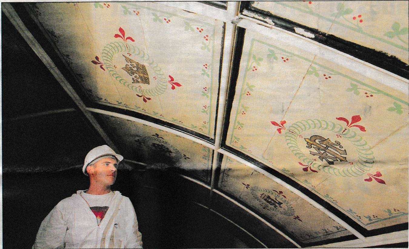
■ HIGHER THINGS: Decorator Joe Reas of Walden and Doyle takes a look at the uncovered panels on St Laurence Church, Stroud's, ceiling.
