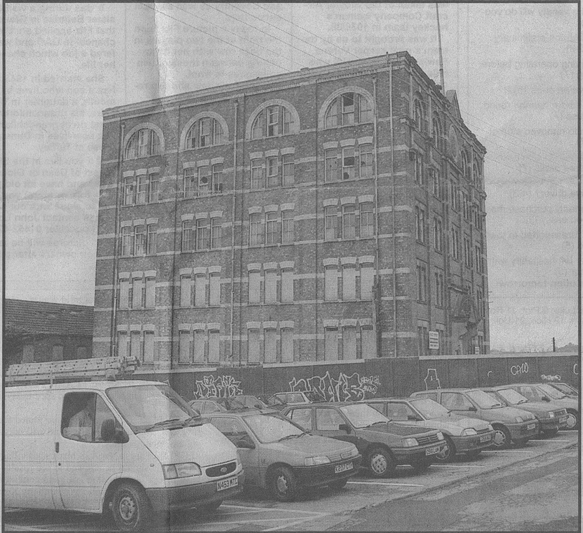
■ The derelict Hill Paul Building which has been the subject of a row between developers and conservationists for years. Demolition contractors moved in today.
